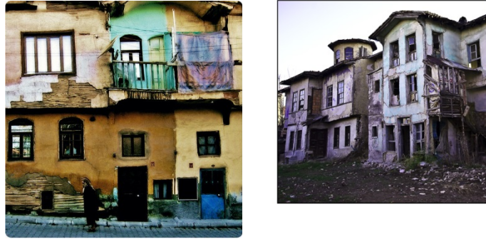
Figure 4: States of the houses in Odunpazarı district before the restoration works Source: http://tr.wikipedia.org/wiki/Odunpazar%C4%B1_Evleri (16.4.2014)
